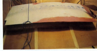
All the windows on the saloon were blown out.
