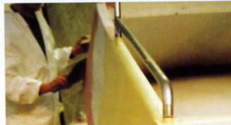
Pitted and bucked steel is faired up with epoxy filler...
